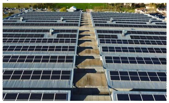
The large photovoltaic system built by Sidel at their Parma plant has become fully operational, enabling the site to satisfy 40% of its electricity needs and cut its CO2 emissions by 871 tons/year, equal to the amount absorbed by 43,500 trees. It is one of the largest corporate photovoltaic systems in Emilia-Romagna, which, thanks to its 5,000 solar panels, is able to produce 2,900 MWh of electricity, equal to the yearly consumption of more than 1,000 Parma households.
